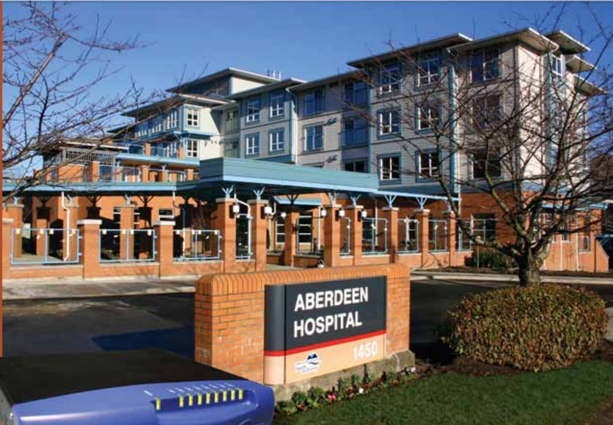
Seniors Housing Centre addition · Victoria, BC
