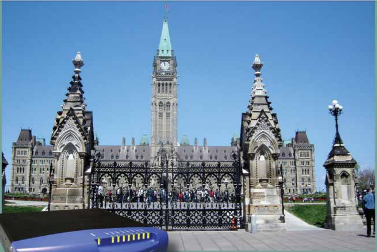
Library of Parliament renovation · Ottawa, Ontario
