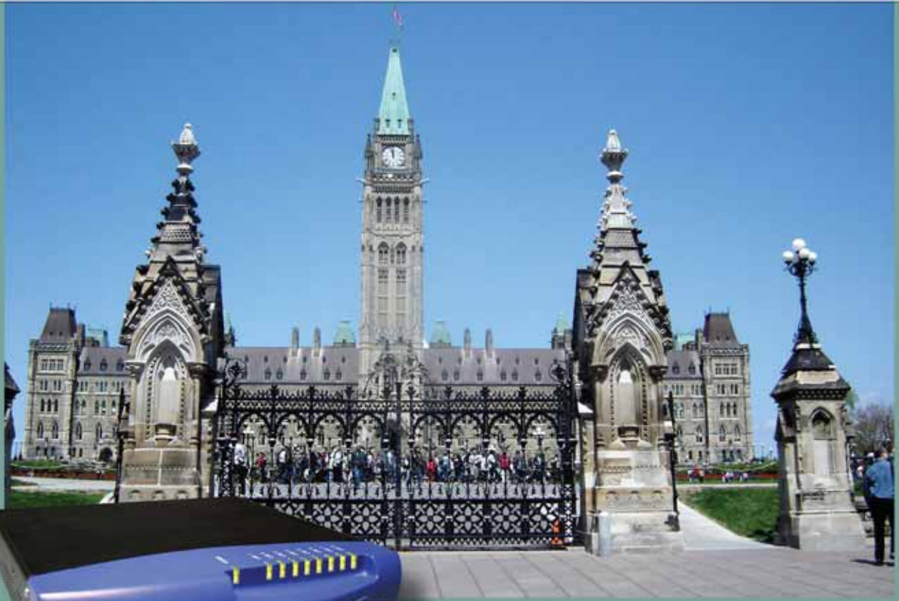
Library of Parliament renovation · Ottawa, Ontario
