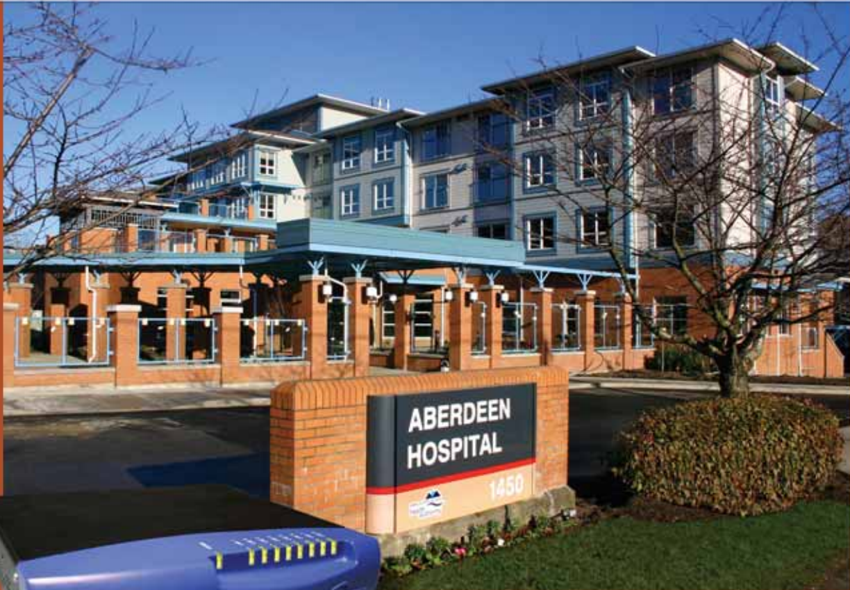
Seniors Housing Centre addition · Victoria, BC
