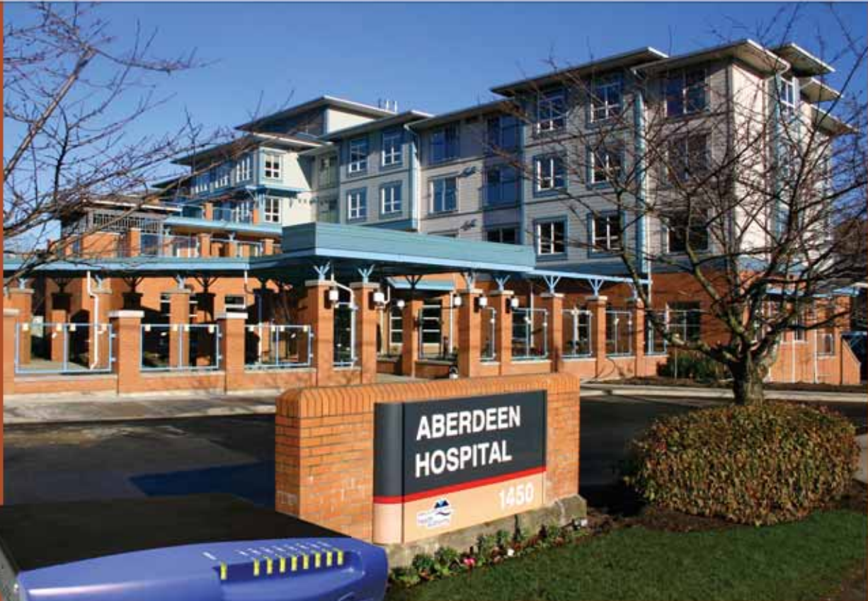
Seniors Housing Centre addition · Victoria, BC
